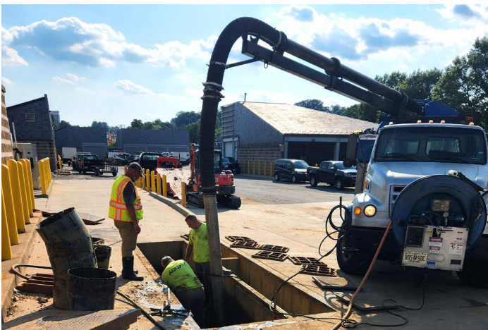
Contractor inspecting and cleaning a stormwater pretreatment chamber at Arlington National Cemetery
